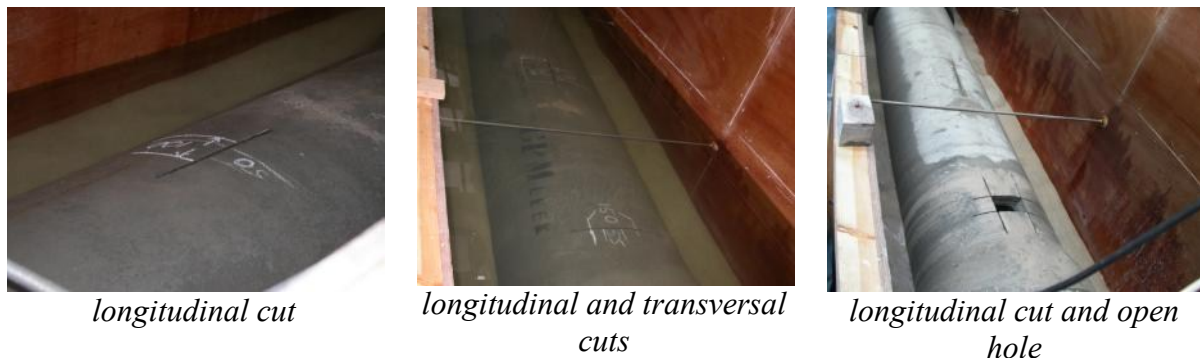
Figure 7. Photographs of the artificial damage inflicted to the top of the horizontal pipe.
